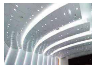
Ceiling curtain wall
